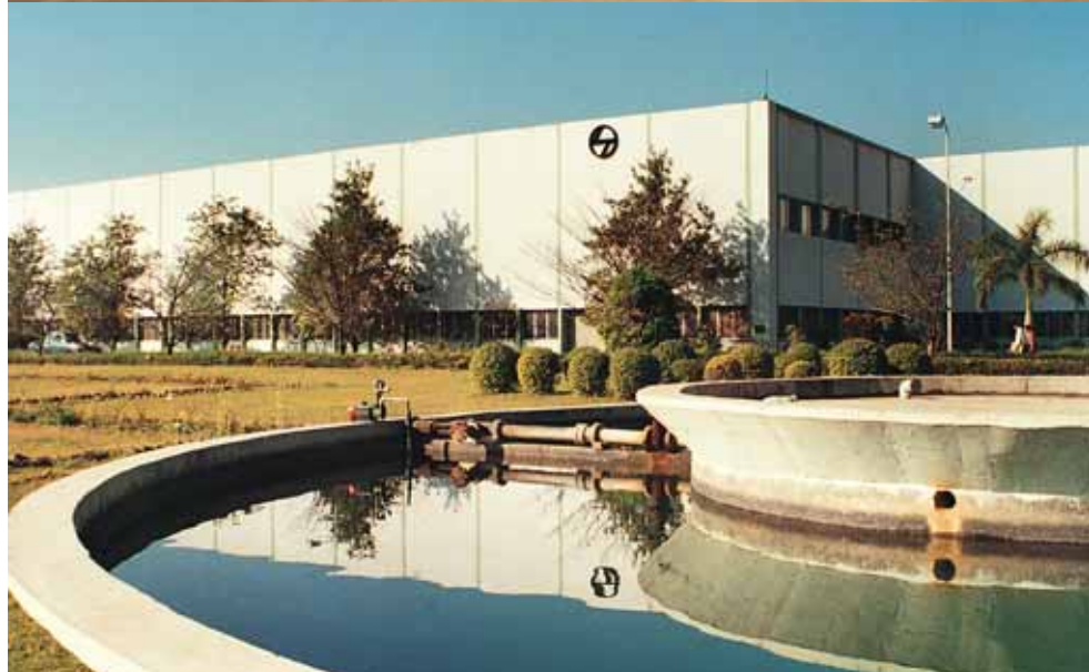
Switchgear Factory, Ahmednagar
