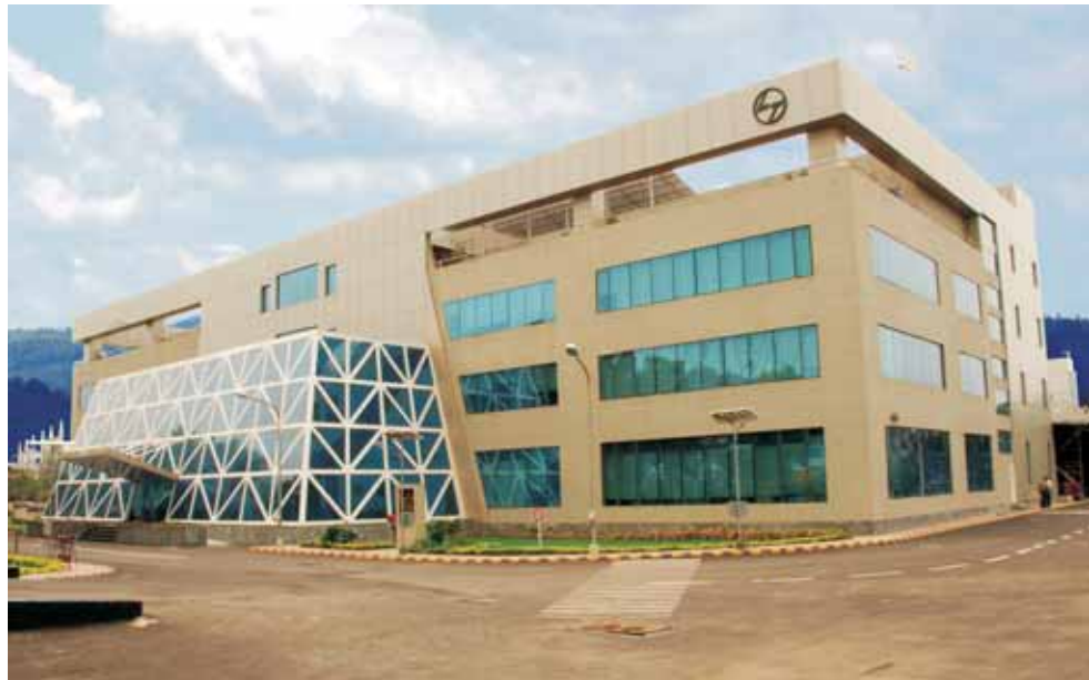
Switchgear Factory, Navi Mumbai
